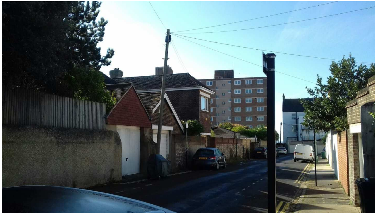
Rear elevation, taken from Westbourne Place, facing South
