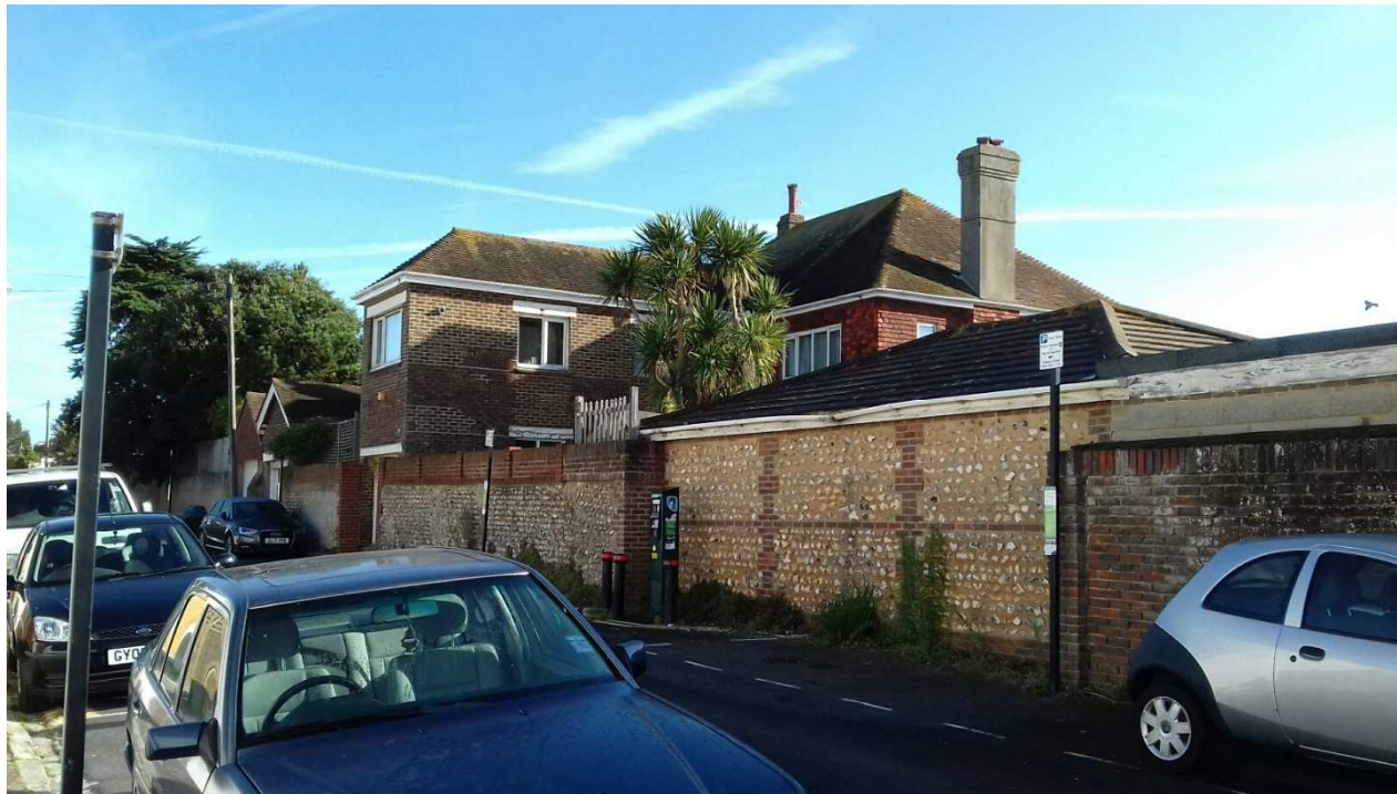
Rear elevation, taken from Westbourne Place, facing North
