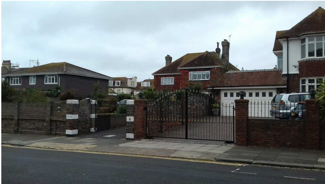
Front elevation, taken from Princes Crescent
