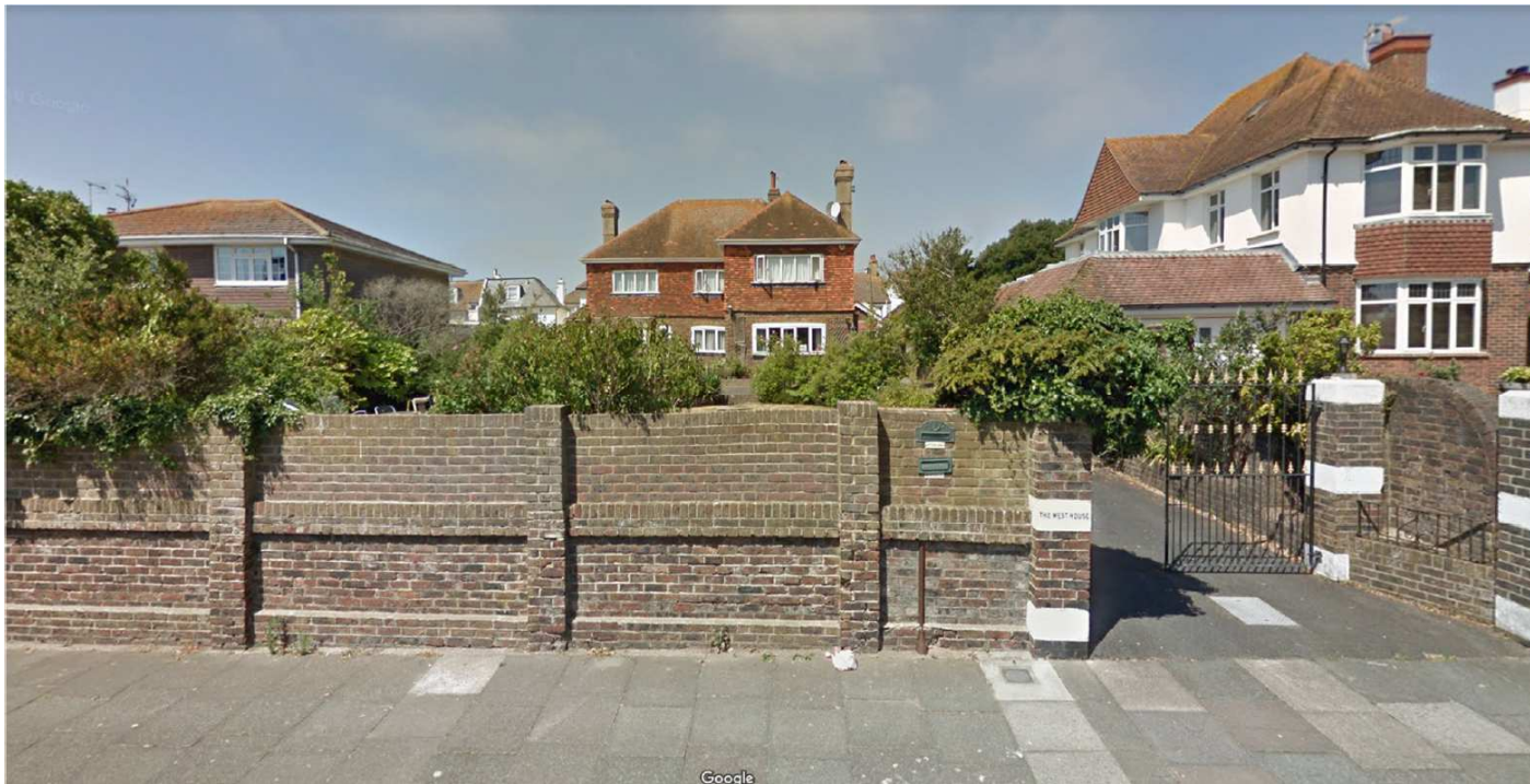
Front elevation, taken from Princes Crescent
