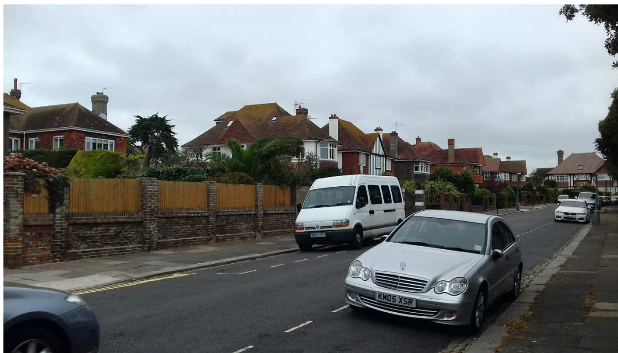
Front elevation, taken from Princes Crescent
